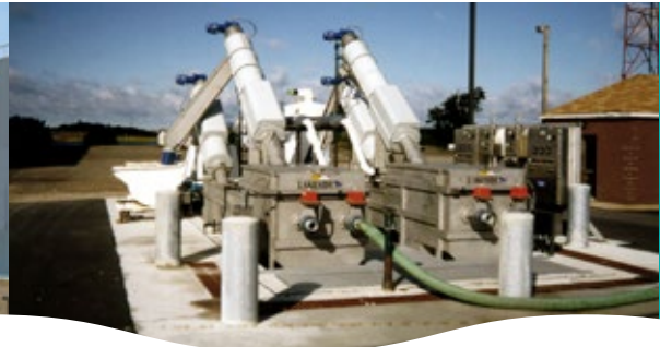
The Complete Plant can be designed with a hook-up for disposal of tankered septage.
