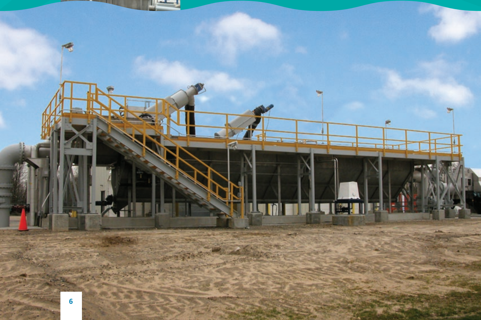
The Raptor® Complete Plant combines screening and grit removal into one self-contained, fully automated unit.
