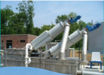
The Raptor® Complete Plant combines screening and grit removal into one self-contained, fully automated unit.
