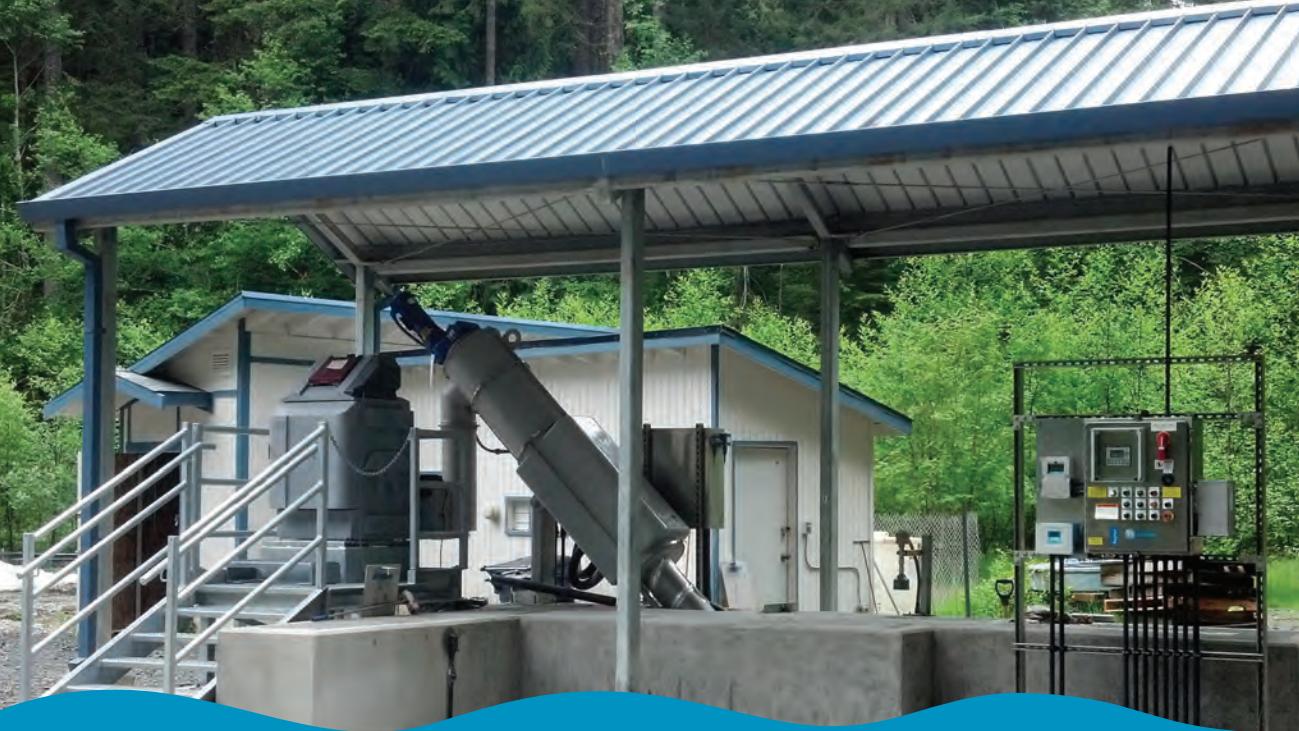
LITTLEROCK, WASHINGTON CEDAR CREEK CORRECTIONS CENTER WWTF
