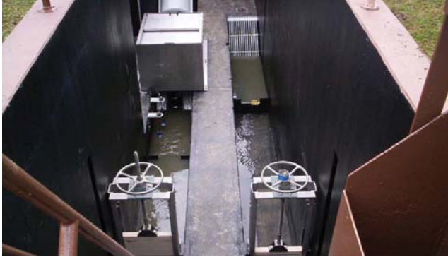
LOOKING INTO THE NEW LAKESIDE RAPTOR SCREEN AT ADDISON
