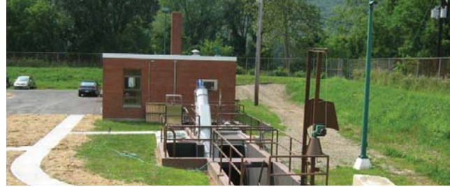
NEW LAKESIDE SPIRAFLO CLARIFIER AT ADDISON
