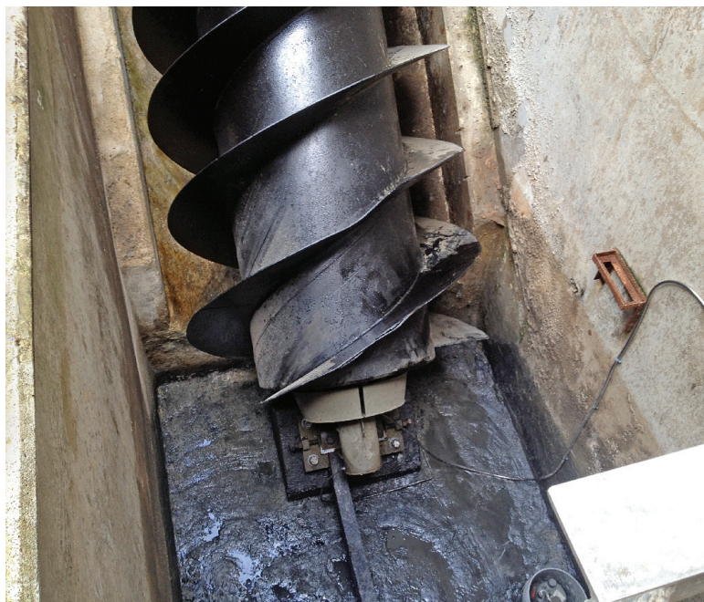
Each pump uses a V-belt drive that protects against possible shock loads.
