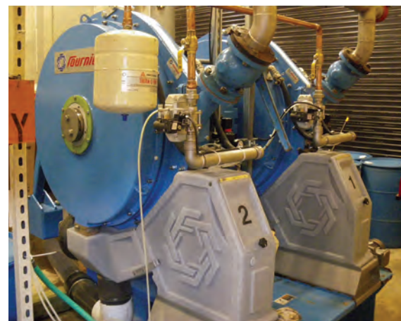
Biosolids are dewatered to 33% solids on this Fournier rotary press.
