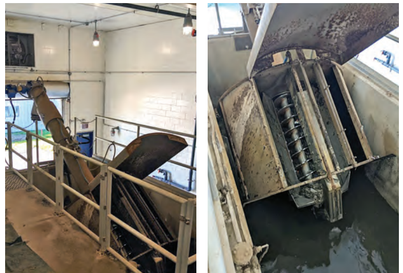
The fine screen’s angled installation and screen bars of varied heights maximize removal efficiency and minimize headloss. It also effectively removes debris such as rags and plastics.
