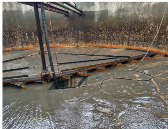
ABOVE: The Lakeside rotors at the Turkey Creek plant sustain high populations of microorganisms. LEFT: Mechanisms in the Lakeside clarifiers move solids to the center for the tank floor.
