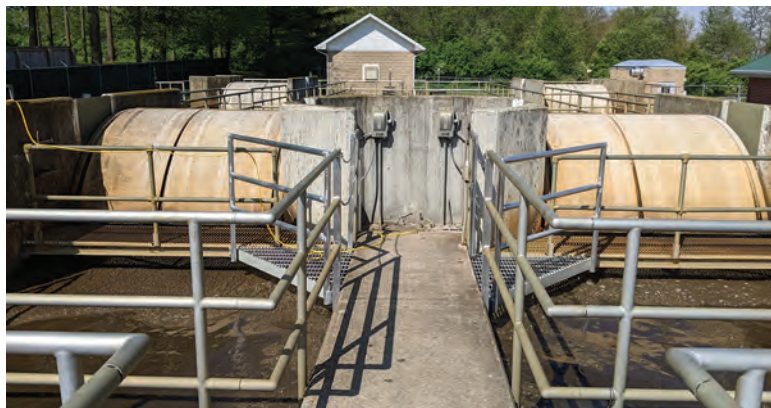
The wide range of oxygen transfer from the rotors enables plant operators to maintain flexibility to match aeration to system demand.
