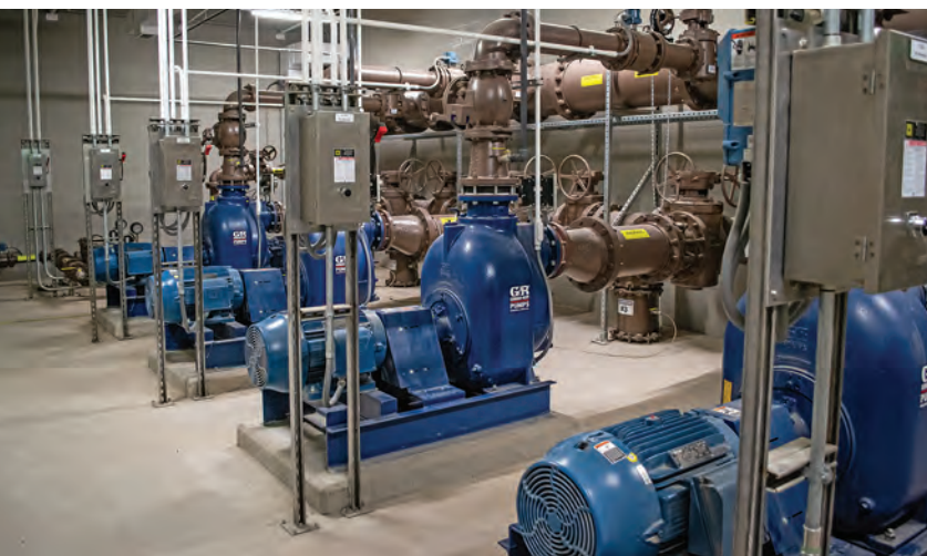
Four Gorman-Rupp pumps convey return activated sludge to the aeration tanks.
