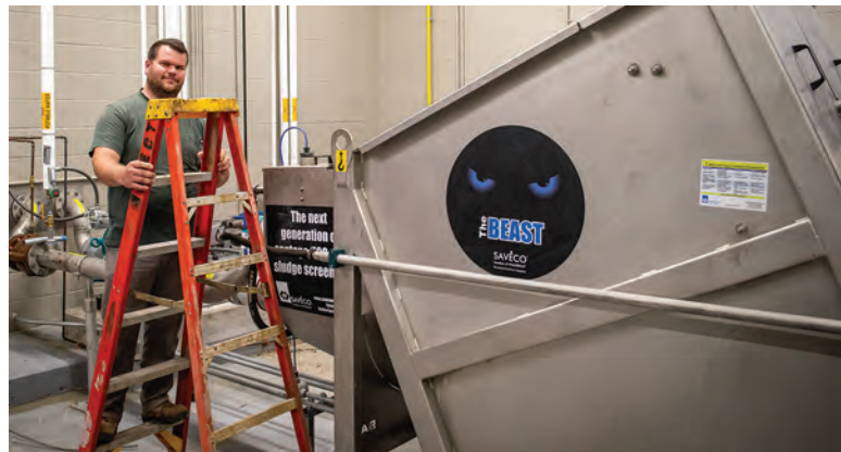
High-strength organic wastes are fed into a pretreatment station (The Beast from SAVECO North America).
