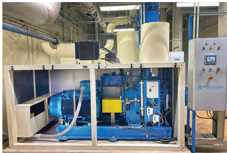
Three single-stage blowers (Continental Blower Industrie) help to automatically modulate flow per the plant’s changing demand, while still maintaining high efficiency.
