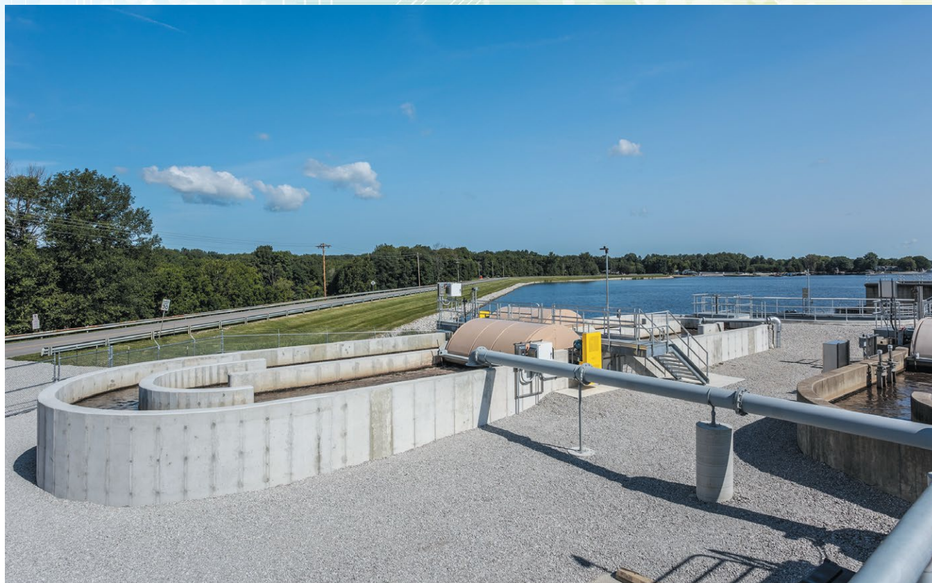
The upgraded Lakeside plant at Heritage Lake benefits from automatic controls which allows the plant to run in storm mode.
