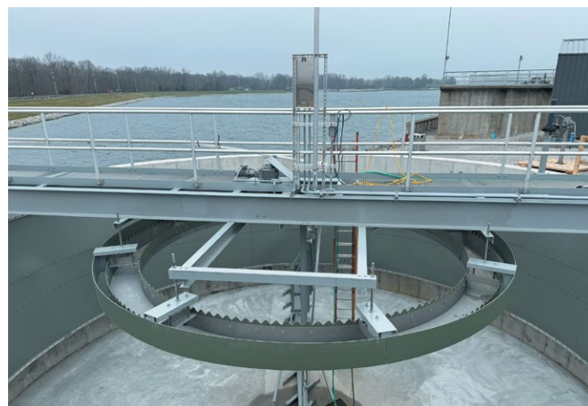
Lakeside's Clarifier removes all types of settleable solids.
