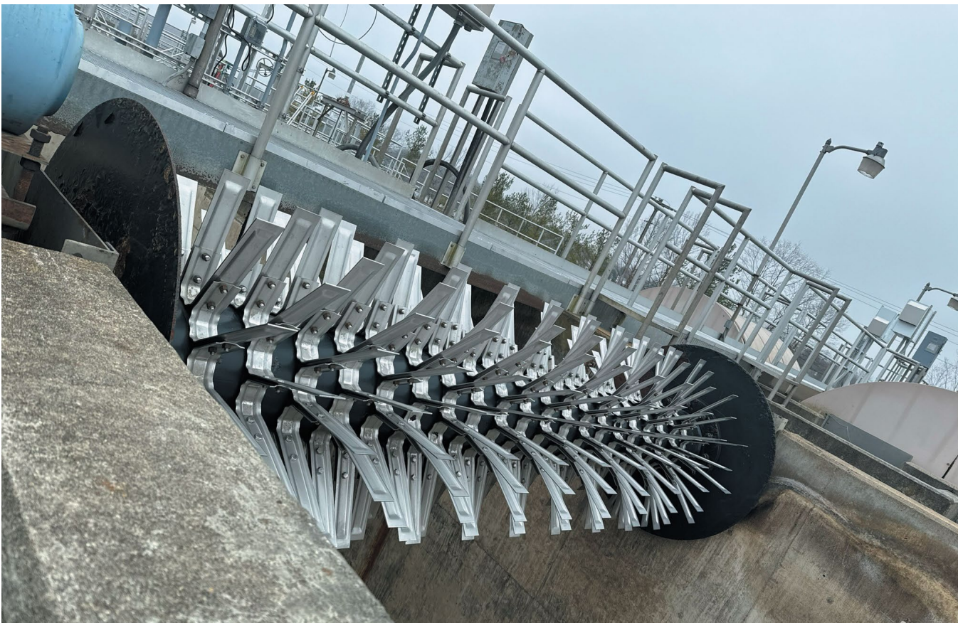
Lakeside's Rotor Aerators provides oxygen to the biological mass and mix microorganisms uniformly to prevent solids from settling in a biological treatment system.
