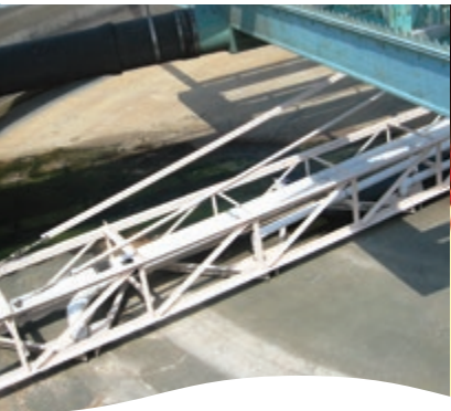
Individual sludge removal pipes in the controlled removal (CR) design
